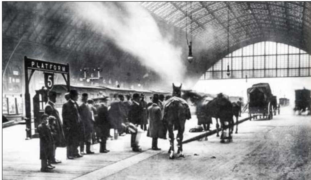
Figure 6.1 St Pancras Railway Station in the 1920s (Source: Carrier, 2012)
