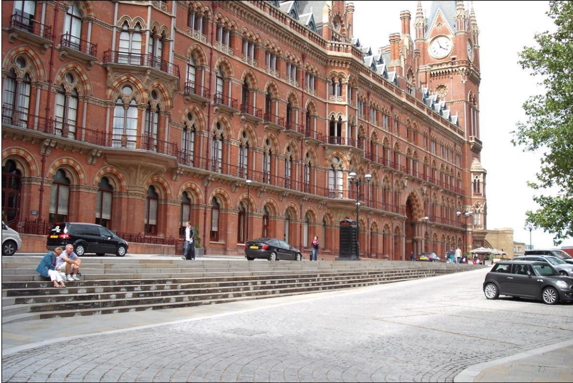
Figure 6.6: Vehicle drop off zone and parking to the front of St Pancras Renaissance Hotel (Euston Road). (Source: Gregson-Green, 2012)
