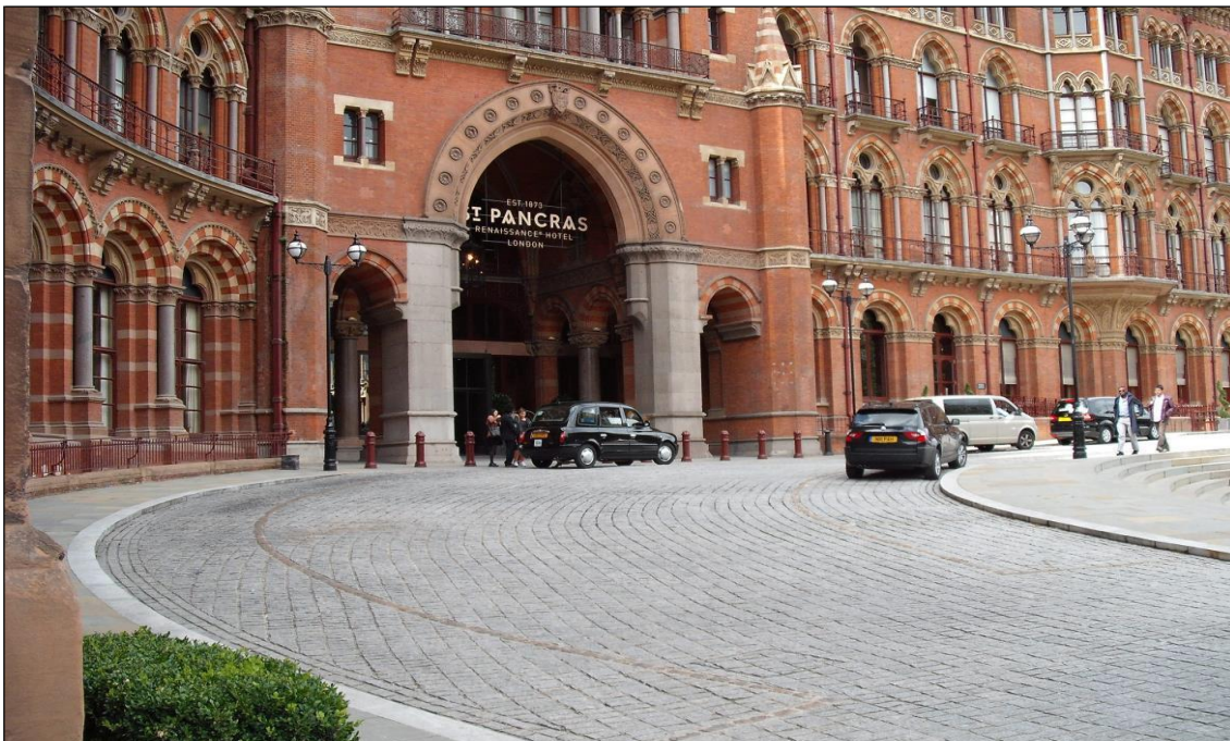
Figure 6.2: Entrance to what was the Midland Grand Hotel, now the St Pancras Renaissance Hotel. Note the hostile vehicle mitigation bollards in front of the entrance, a heritage design to be in keeping with the exterior of the hotel. (Source: Gregson-Green, 2012)
