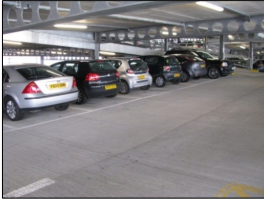
Figure 6.5 Multi storey car park
