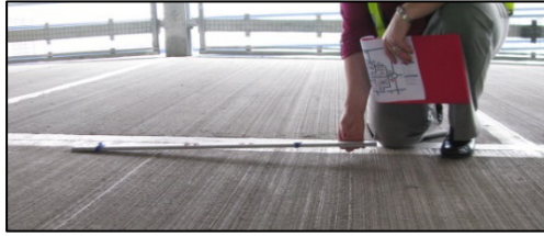
Figure 6.2 Measuring the gradient
