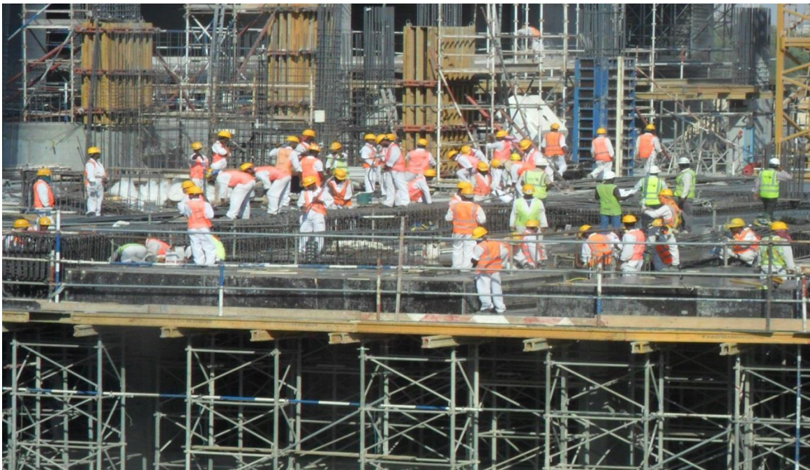
Picture 2.3 Construction workers in Dubai
