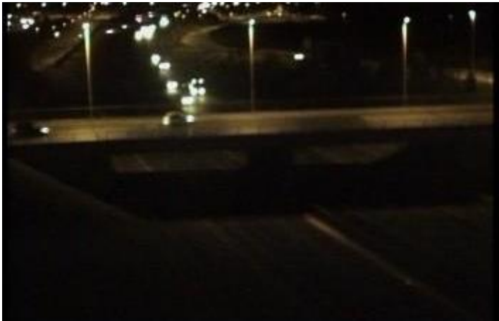
Figure 3.1 M1 Northbound Motorway, Junction 46, Leeds – visibility problems at night-time
