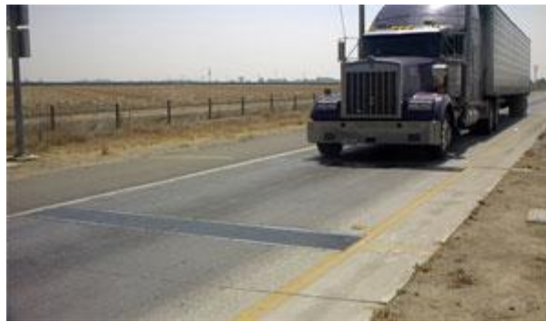
Figure 3.4 Bending plate WIM system (Source: International Road Dynamics, Inc.)
