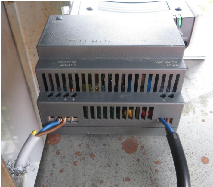
Figure C8 Power switch of the radar system installed on the M1-A1 Link Road
