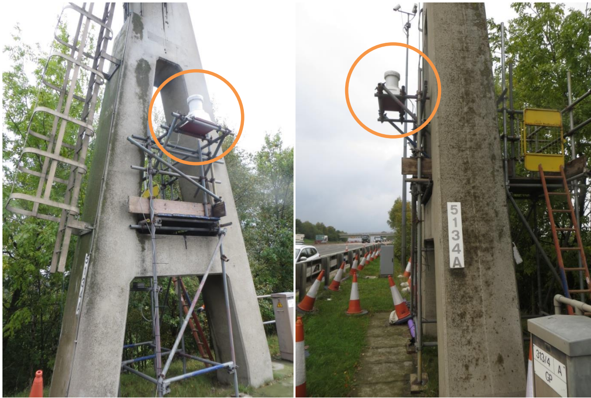
Figure C3 The scaffold installed on the M1-A1 Link road for the radar mounting
