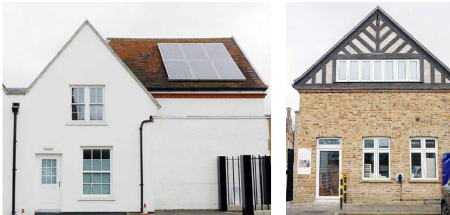
Fig. 4. Victorian semi-detached house, with side view
