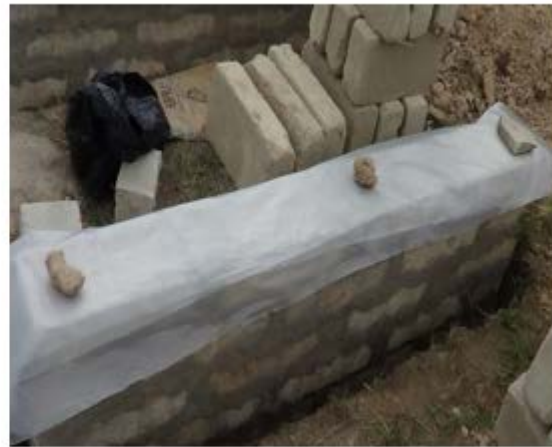
249 Fig 2 (a) Schematic diagram of the position of the dpc (b) Photograph showing how the dpc was 250 laid (Source: Agyekum et al., 2016)
