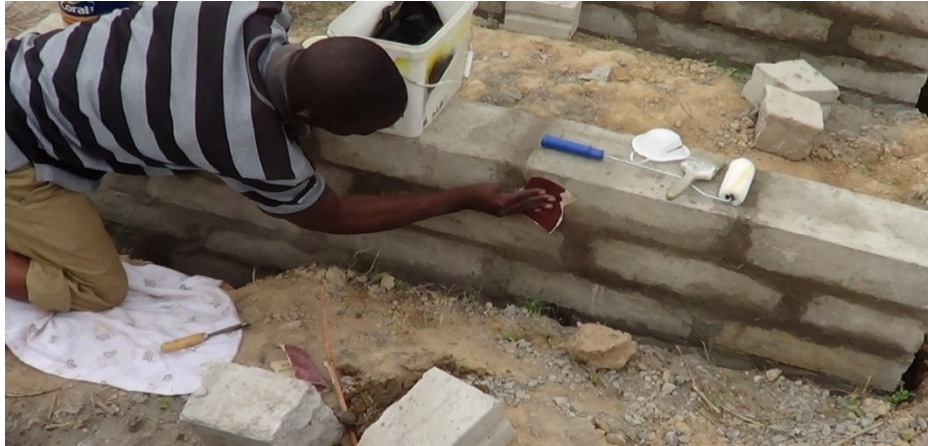
Fig 4 Photograph showing the preparation of the wall surfaces
