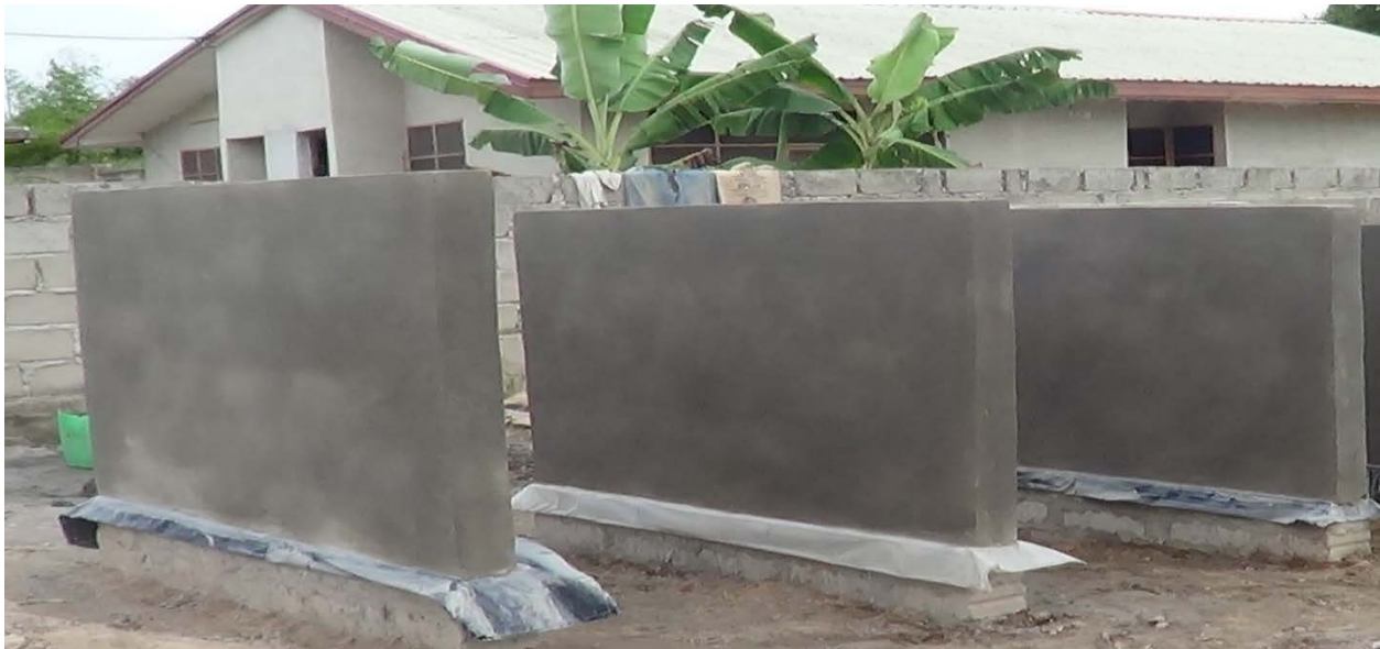
251 252 Fig 3 Photograph of test walls after the dpcs were laid
