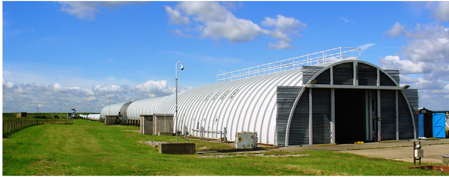
Fig. 1. The Air Blast Tunnel (ABT), MOD Shoeburyness, UK (Clubley, 2013).
