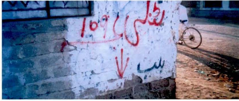
Sector 11½, Orangi Town; view of tank
