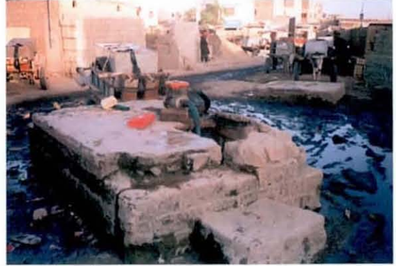
Illegal water supply from an existing conduit – water venders are benefiting from its operations
