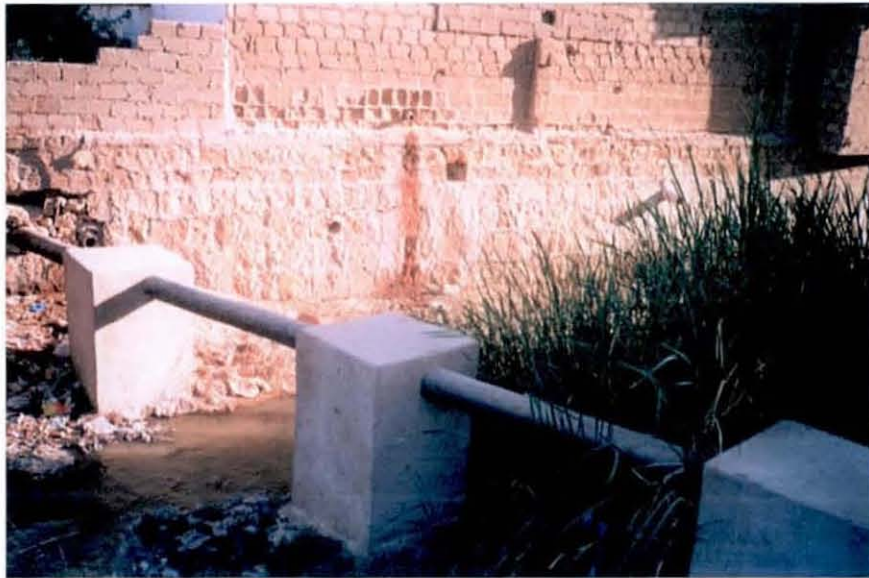
Water line passing through the nullah
