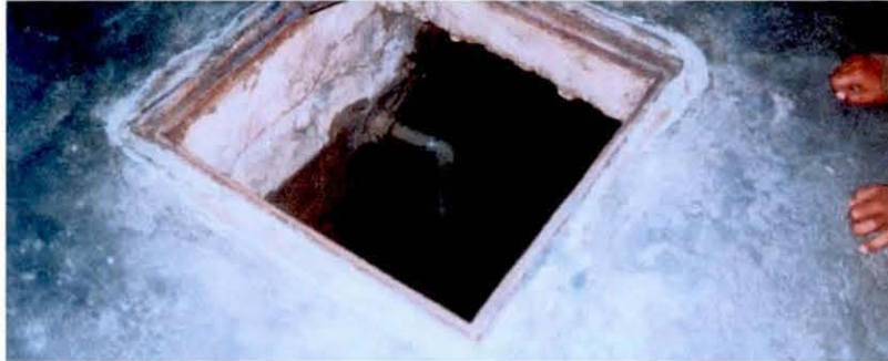
Orangi Town: Internal view of tank no. 3
