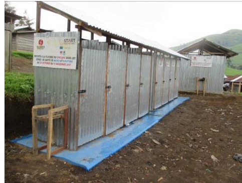
Photograph 2. Latrines completed in Rubaya
