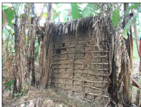
Photograph 3. A traditional pit latrine constructed using low-cost materials
