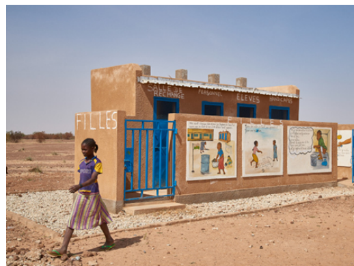
Photograph 6. Latrines built by the project
