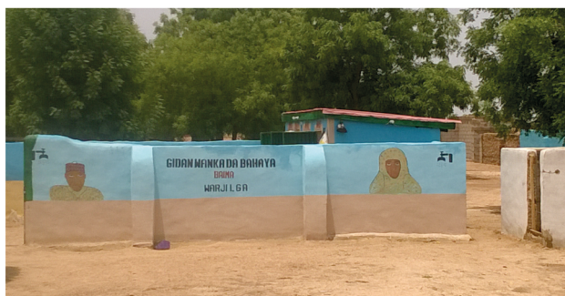
Photograph 1. Facility constructed through PPP at Bama Market, Warji LGA, Bauchi State
