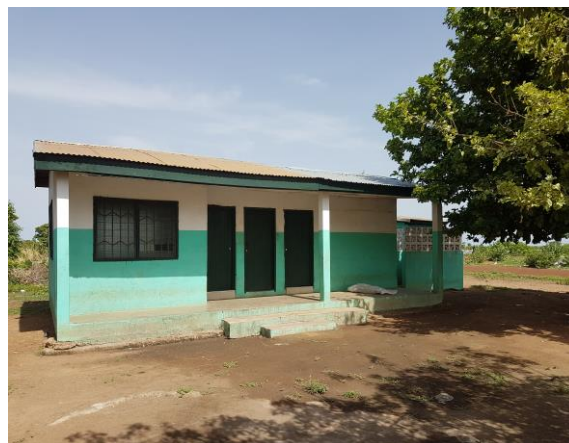
Plate 4.12: WMA's waste disposal site office (1:100cm scale)
