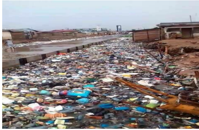
Plate 1: A choked drain in Accra, Ghana, after a rain
