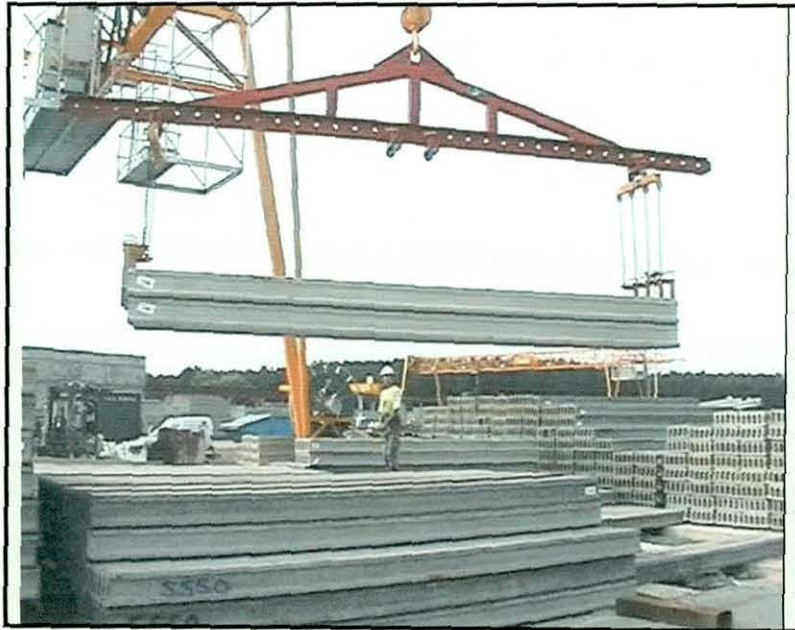
Figure 4.5 Precast flooring (hollowcore) stockyards - Courtesy of BPCF (2005).
