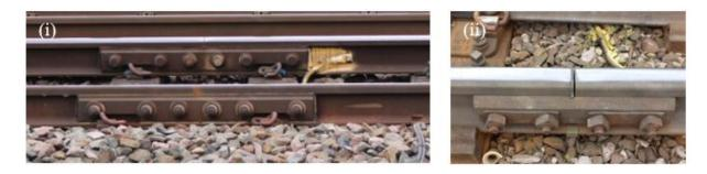
Figure 1.7 (i) 6-bolt and (ii) 4-bolt rail joints in UK site 2015 (Author's personal collection)
