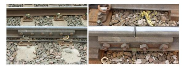
Figure 2.12 (i) A glued 6-bolt IRJ and (ii) a dry 4-bolt IRJ
