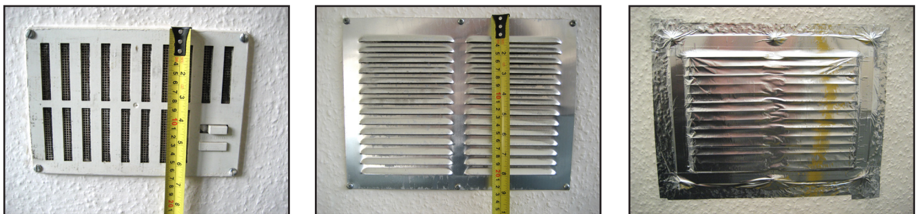
Figure 5. Fireplace vents sealed with aluminium tape to ensure uniformity between houses.
