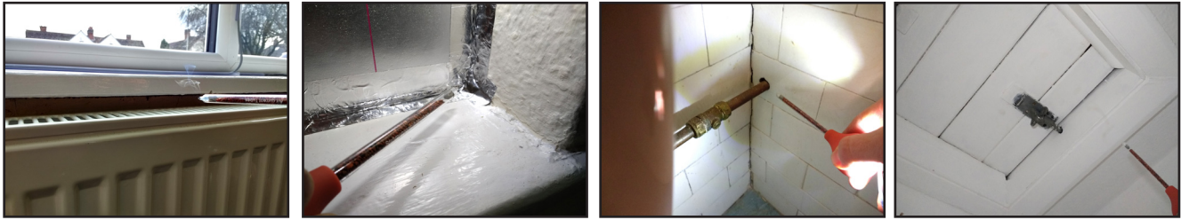
Figure 7. Qualitative air leakage testing using smoke sticks.
