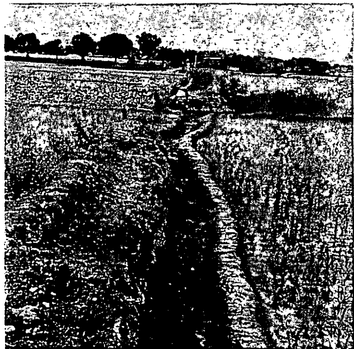
TADP (Bangladesh) Field channel alongside previous raised distribution channel
