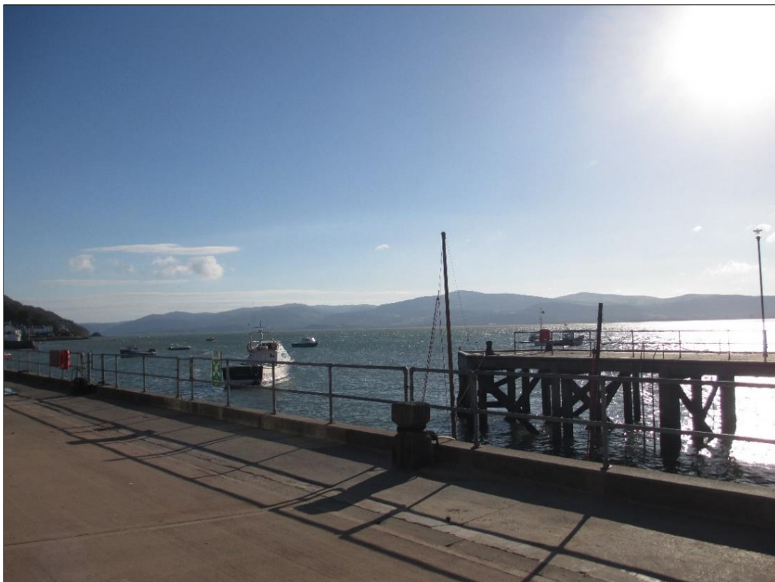
Figure 3.3 The wharf at Aberdovey, showing the jetty on the right-hand side (authors own photograph)
