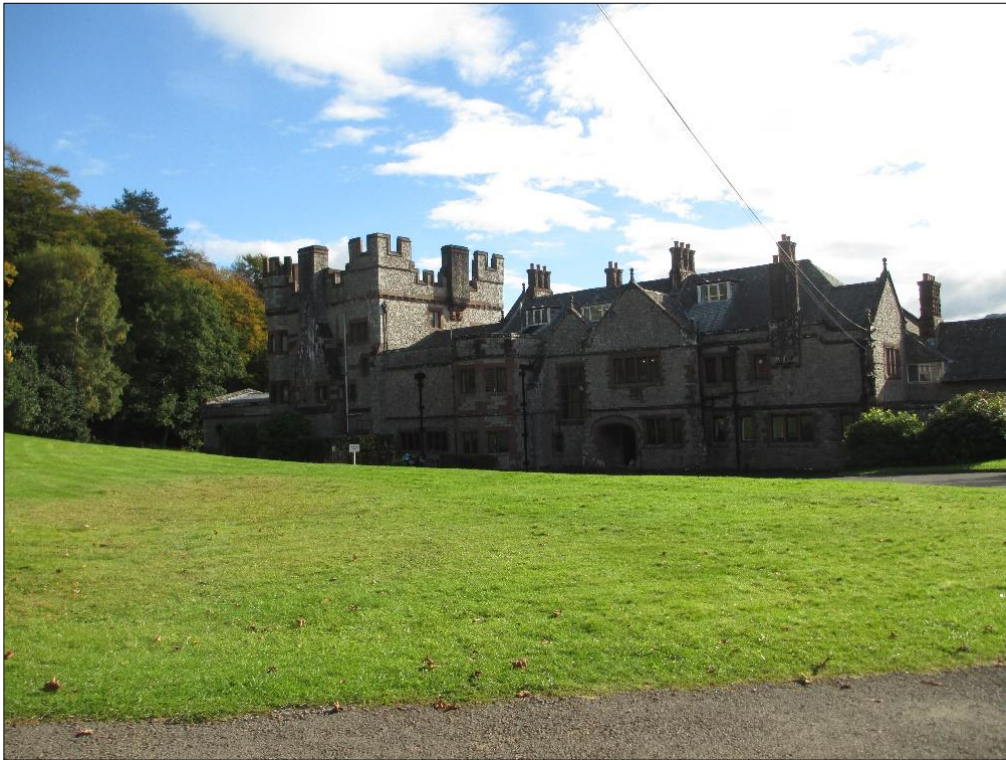
Figure 4. 1 The main building at Eskdale (authors own photograph)
