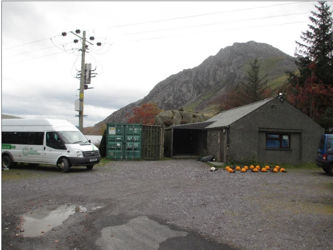
Figure 3. 4 The stores at Ogwen Cottage (authors own photograph)
