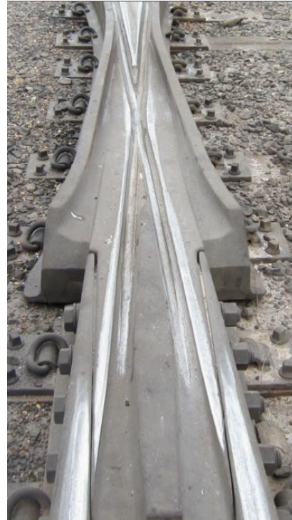
Figure 2.13: Flange bearing crossing nose [13]
