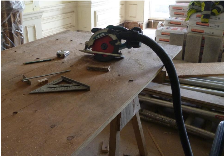
Figure 2 Once workers become used to working with on tool dust extraction, they are more likely to use it by choice on future jobs
