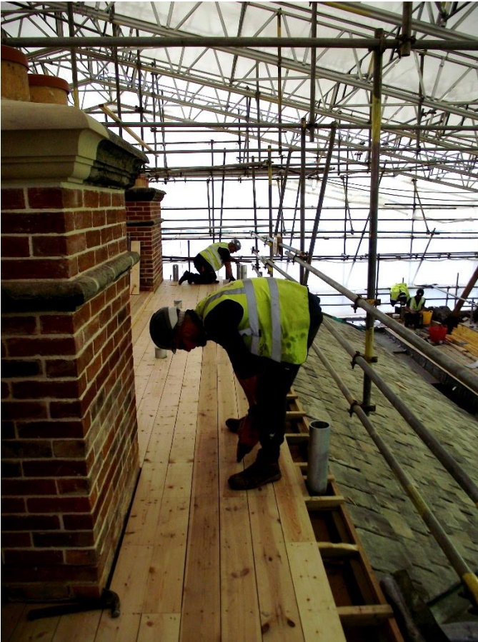
Figure 3 Manual handling and poor working postures are an ongoing challenge in construction
