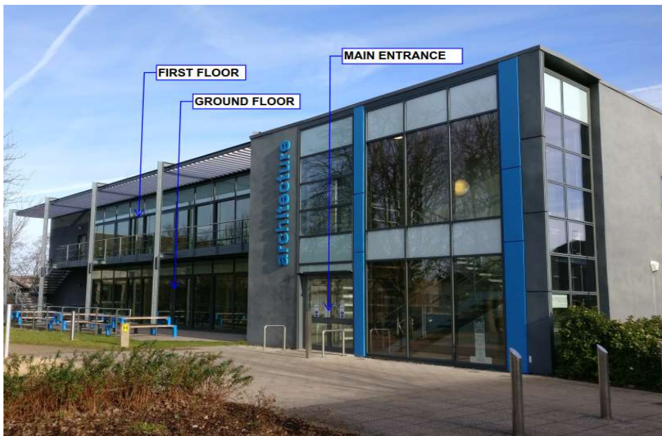
Figure 5 - School of Architecture - Keith Green Building, Loughborough University
