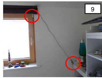
Figure 3-52- State logger & window sensor – From left to right - located on the tilt & turn window in bedroom 3 and bedroom 4 (source: author)
