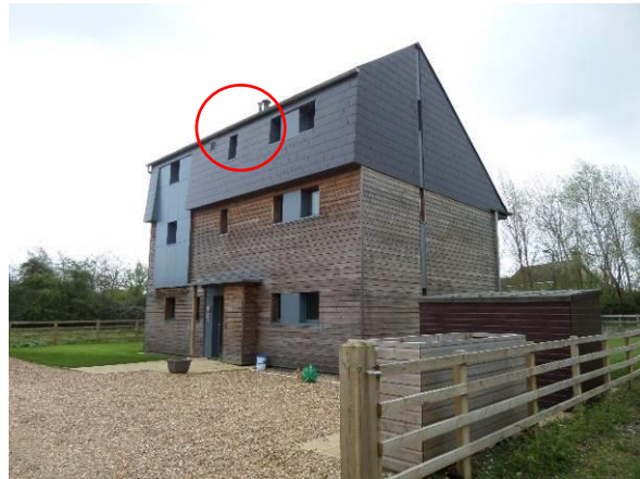
Figure 4-39- Rear elevation (northeast) indicating the location of the extract through the roof and the fresh air through the wall (highlighted in red) (source: author)
