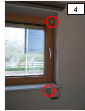
Figure 3-43- State logger & window sensor - From left to right located on the tilt & slide window in the dining room, living room, kitchen and study area (source: author)
