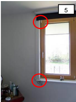
Figure 3-48- State logger & window sensor - From left to right - located on the tilt & turn window in the main bedroom, bedroom and master bathroom (source: author)
