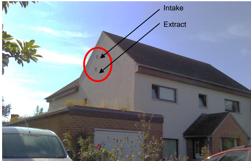
Figure 4-57- Northeast façade indicating the position of the MVHR extract and intake, extract is located below the intake on the wall.
