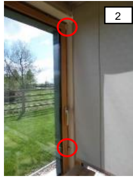
Figure 3-43- State logger & window sensor - From left to right located on the tilt & slide window in the dining room, living room, kitchen and study area (source: author)
