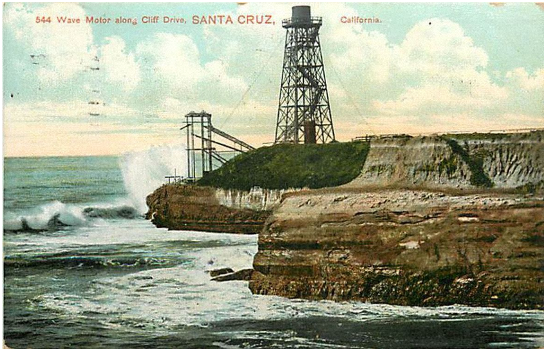
Figure 1.2: Postcard of the Armstrong brothers' Wave motor. It functioned from 1898 to 1910 in Santa Cruz, CA. [35].
