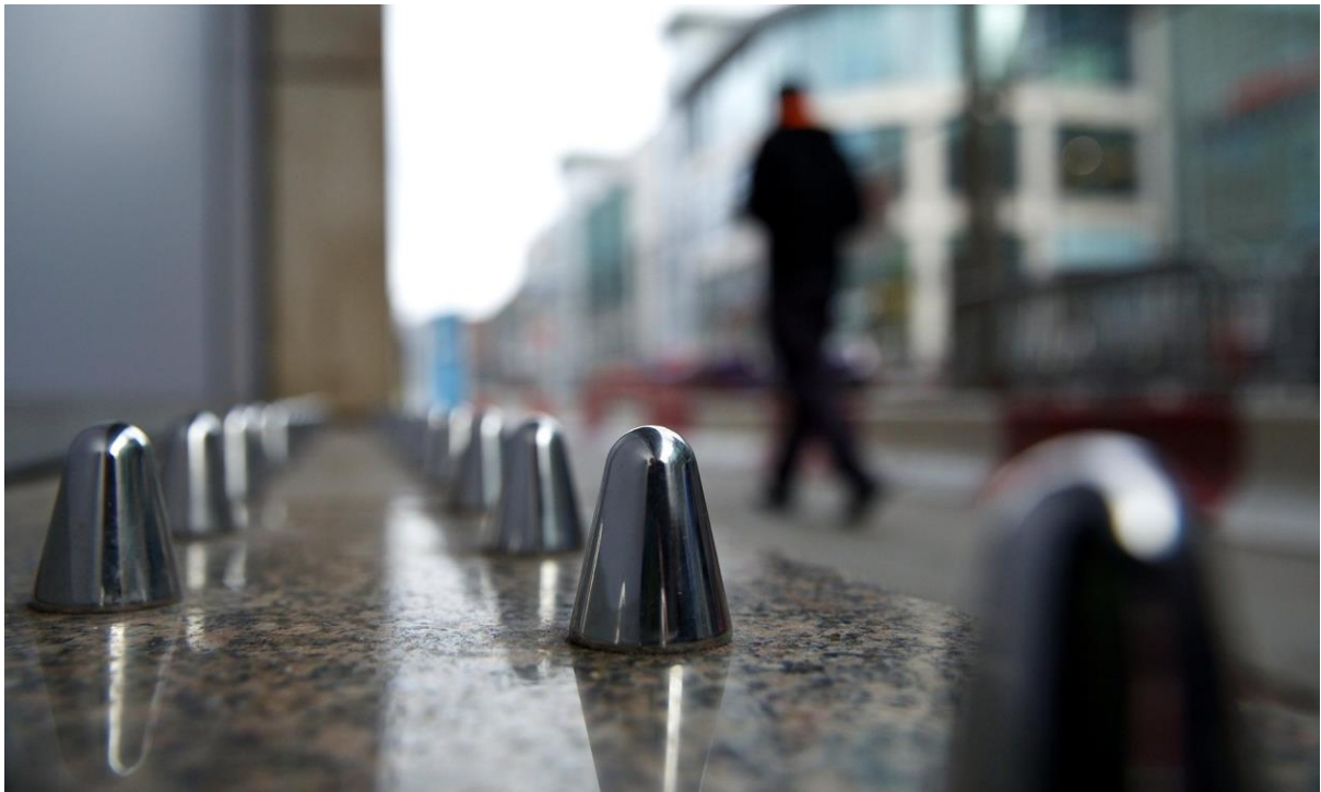
Figure 28 Spikes outside Selfridges in Manchester (photo taken by Christopher Thomond for the Guardian - https://www.theguardian.com/society/2015/feb/18/defensive-architecture-keeps-poverty-undeen-and-makes-us-more-hostile#img-4
