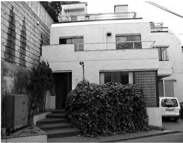
Figure 9. c-MA1, exterior: before (Sources: IKDS)
