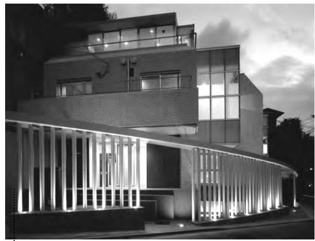
Figure 10. c-MA1, exterior: after (Sources: IKDS)
