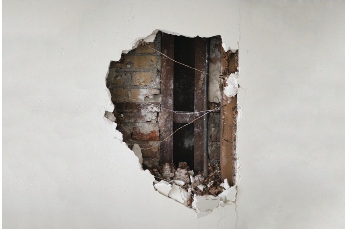
Fig. 6 : Vertical stratigraphy from the work site Les Petites Affiches (2018) - © Anna Saint Pierre
