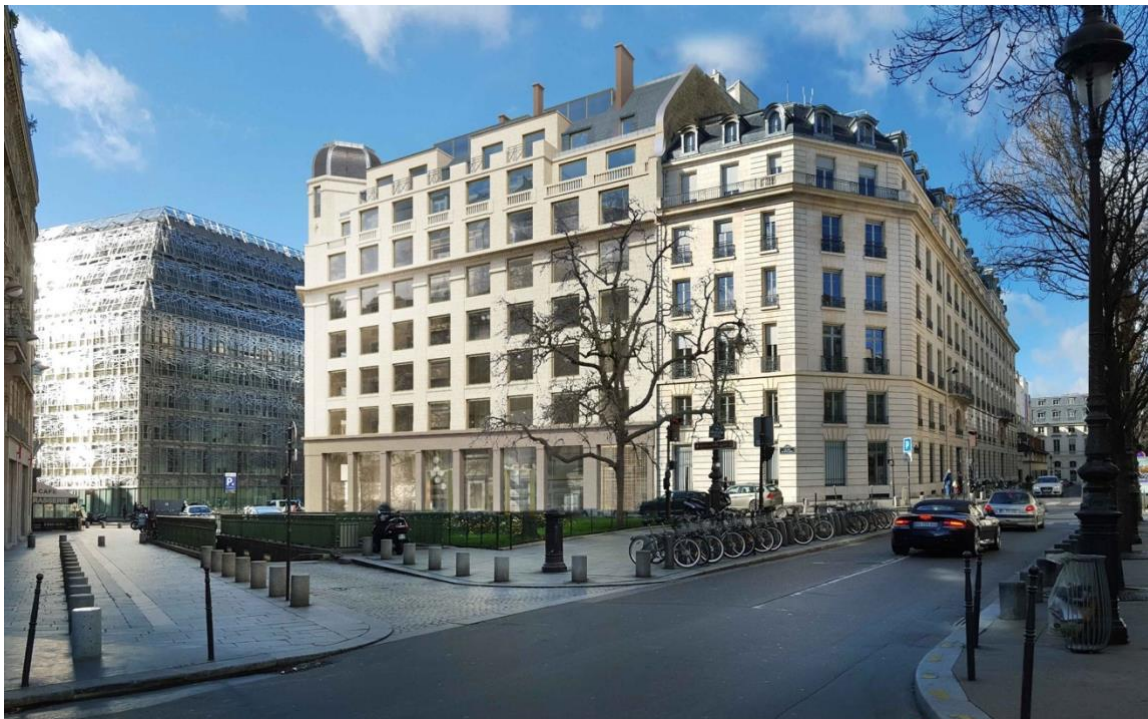
Fig. 9 : Images of the project - © SCAU architecture
