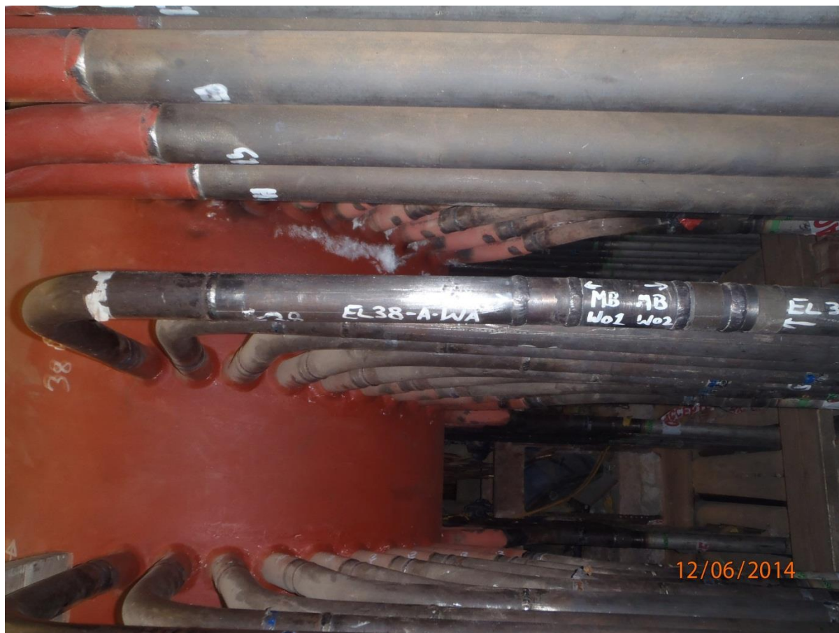
Figure 9.8: A photograph showing a section of MarBN material installed within an operating coal fired power plant in June 2014, Photograph Courtesy of Dr C.Degnan, EON
