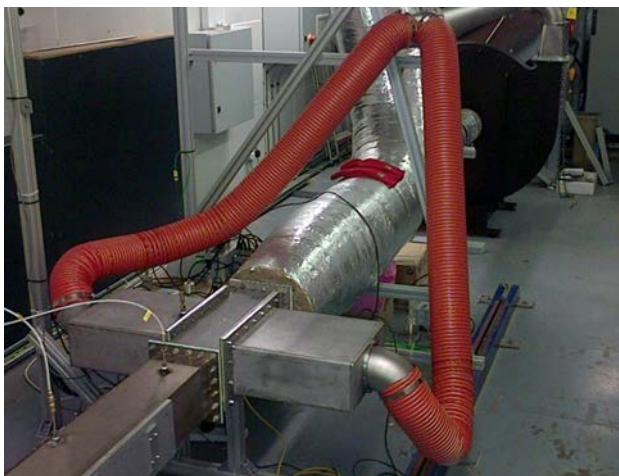
Figure 28 –Turbulence Generator prior to installation of insulation
