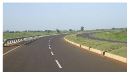
Fig. 4.13: MP1 Highway, India
