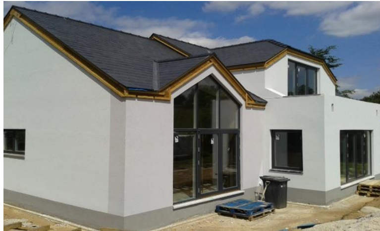
Figure 4 South-West view of the building case study
