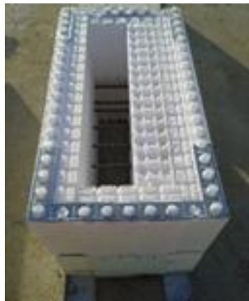
Figure 1 Prefabricated Expanded Polystyrene (EPS) hollow block of ICF, before the concrete is poured.
