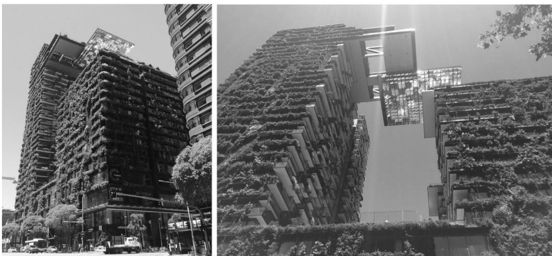
Figure 6-17: The Heliostat, Central Park. Landmark building with a green façade. Photographs by author.
