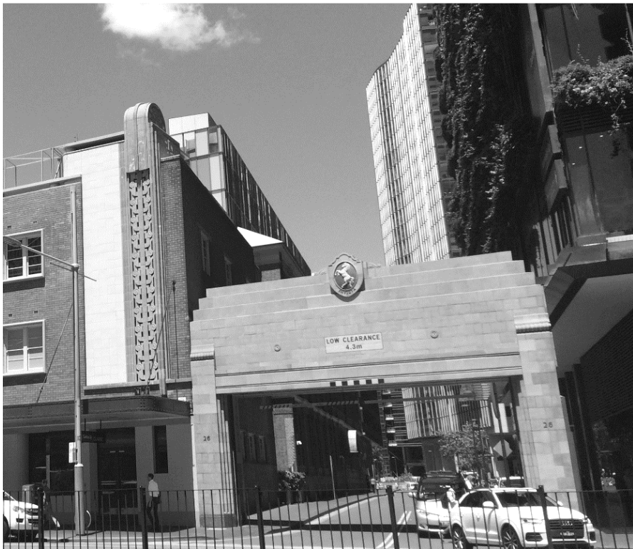
Figure 6-8: Retained portal gate for former brewery, Central Park. Photograph by author.
