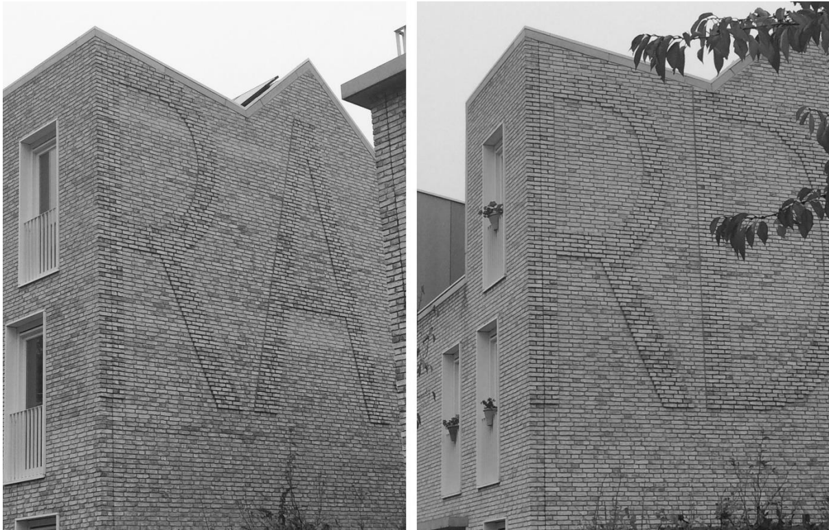
Figure 6-18: Lettering in relief of brickwork on Strijp-R's new build housing. Letters represent name of building that was demolished in that location. Photographs by author
