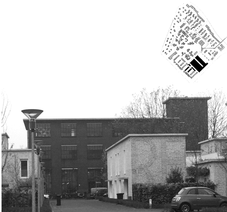
Figure 5-17: Juxtaposition of scales on Strijp-R. Retained industrial building alongside smaller scale new build residential housing. Photograph by author.
