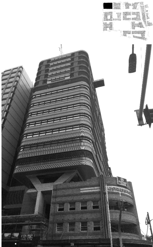
Figure 5-16: Juxtaposition of scales on Central Park. Retained pub with new building cantilevering over the top. Photograph by author.
