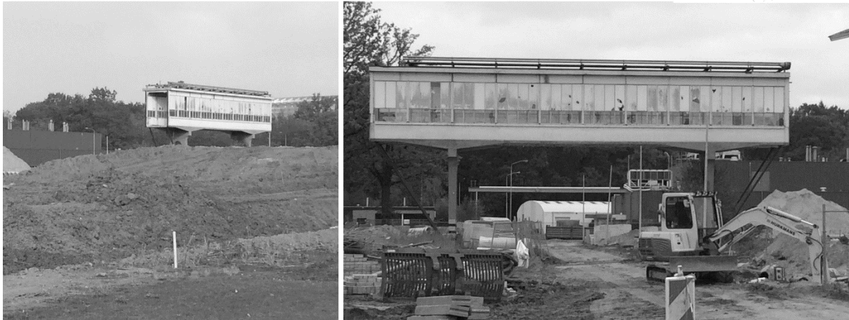
Figure 5-18: Retained walkway, Strijp-R. Photograph by author.
