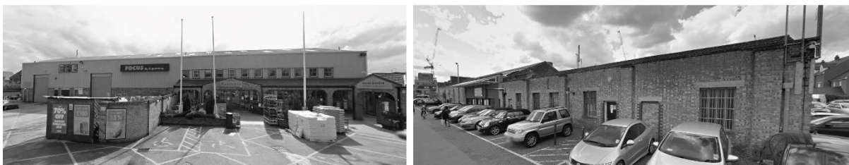
Figure 5-8: Demolished buildings on the 'Northern Sidings', CB1. Demolished due to poor quality. Image source: Google Street View, CB1.
