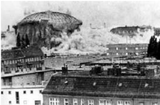
Figure 4. Demolition of the Gasometer. Photo : Prenzlauer Berg Museum
