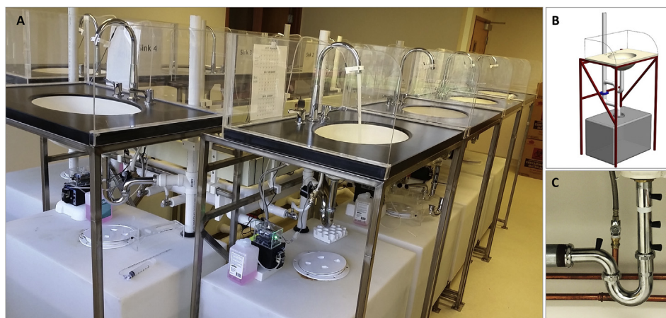
Fig. 1. A) Sink lab infrastructure with an array of nine modular sink rigs operated using indigenously developed automation; B) schematic of a single sink module; C) Sink plumbing depicting the sampling ports [*] for P-trap water and biofilm sampling.
