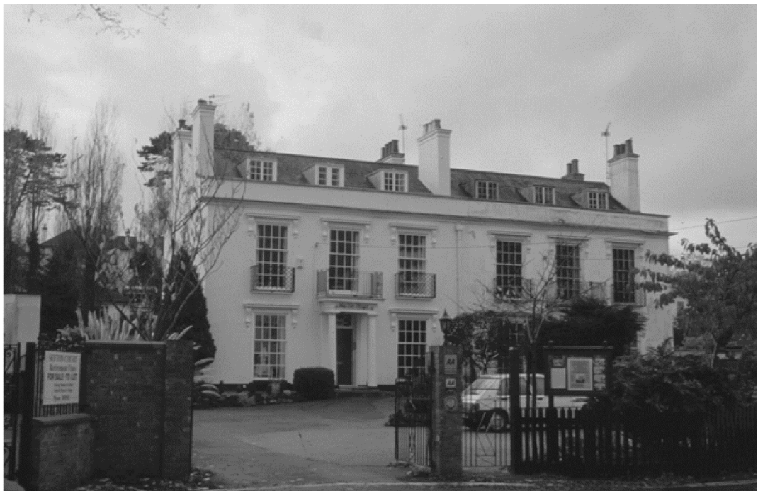
Figure 1.7: Late Georgian cob town houses in Dawlish, Devon, built c. 1820 (from Keefe, 2012).
