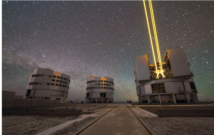
Figure 2.19: Photograph of the four sodium LGSs used by the AOF on the 8.2m Yepun telescope at the VLT, Paranal (Horálek, 2018).
