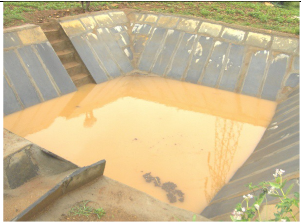
Farm Pond lined with cuddapah slabs
