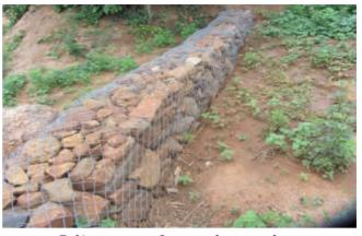
Gabion structure for groundwater recharge
