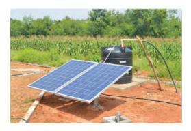
A small scale solar powered micro-irrigation system was designed and installed for the demonstration and use of small farmers having <=1 acre land under IFS module for growing vegetables under farm pond system.
