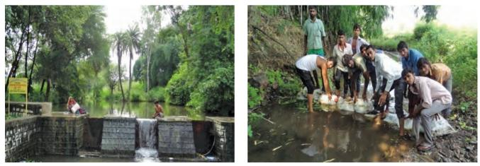
Renovated water harvesting structure with water, polybag check dam and soybean crop in Jhabua, M.P
