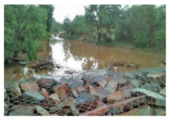
Rainwater harvesting through gabion check dam for ground water recharge
