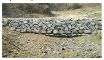
HDPE film embeded Gabion checkdams
