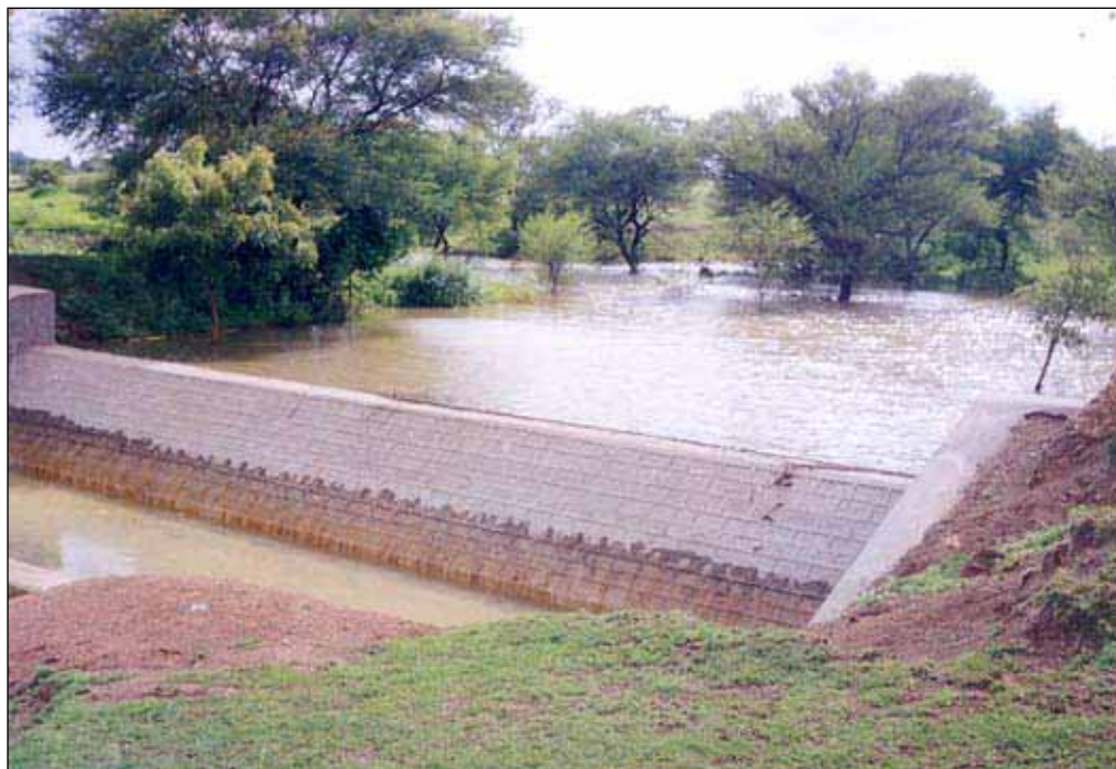
Figure 4. Water stored in check dam built across the stream channel (ex-situ management); Photo: Kothapally watershed.
