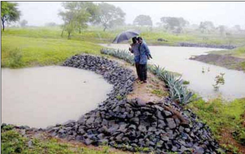
Figure 1. Water harvesting structure in Adarsha watershed Kothapally, Andhra Pradesh.
