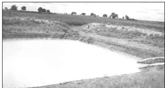
Farm pond at Joladarasi watershed showing inlet, outlet and spoil bank
