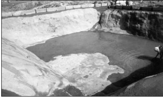
Farm pond lined with cement + soil (1:8)
