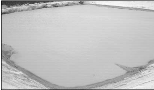
Farm pond lined with cement + murrum (1:6)
