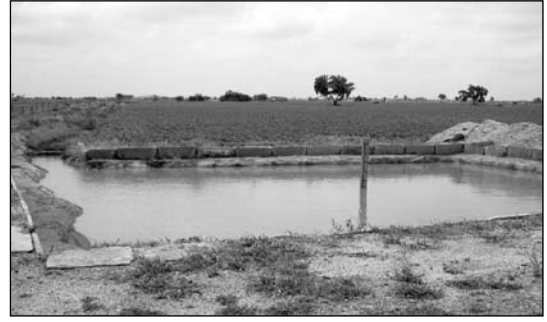
Farm pond lined with cement + soil (1:8)
