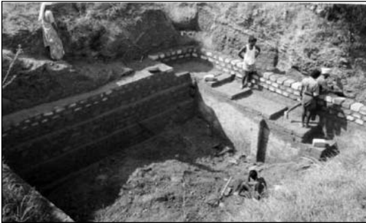
Farm pond lined with cement bricks
