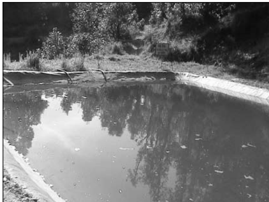
Figure 1 and 2. LDPE sheet water storage pond at UHF Nauni, Solan.
