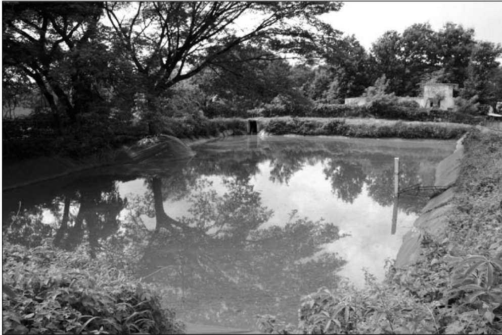
View of a larger farm pond lined with 300 GSM silpaulin poly films
