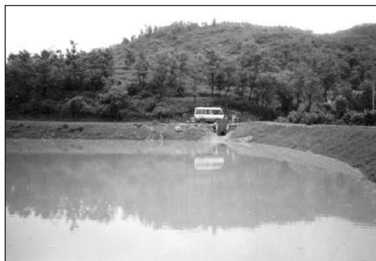
Multi purpose check dam for harvesting surface and sub-surface water and diverting to main pond
