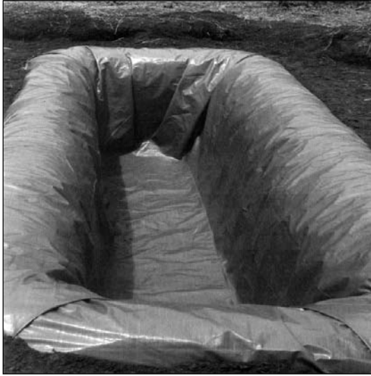
Lining of a smaller farm pond with 200 GSM Silpaulin poly film
