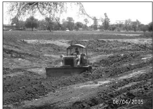
Use of Bulldozer
