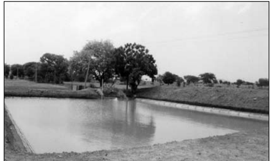
Farm pond lined with Kadapa slabs
