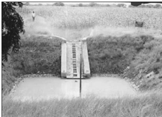
Farm pond – Grassed waterway leading to farm pond (inlet, gauging scale seen)
