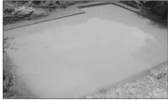
Farm pond lined with cement bricks
