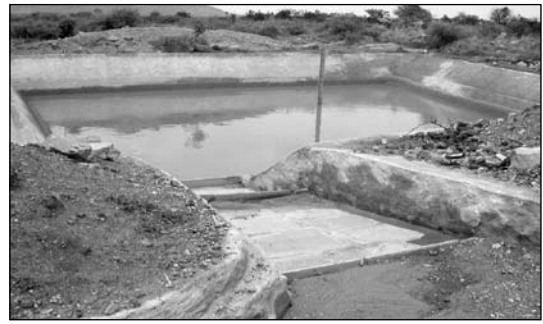
Farm pond lined with bricks
