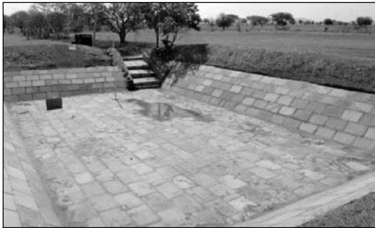
Farm pond lined with Kadapa slabs
