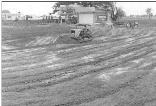
Use of Bulldozer
