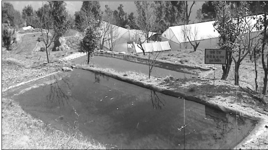
Figure 6. LDPE lined water storage demonstration by VPKAS, Almora
