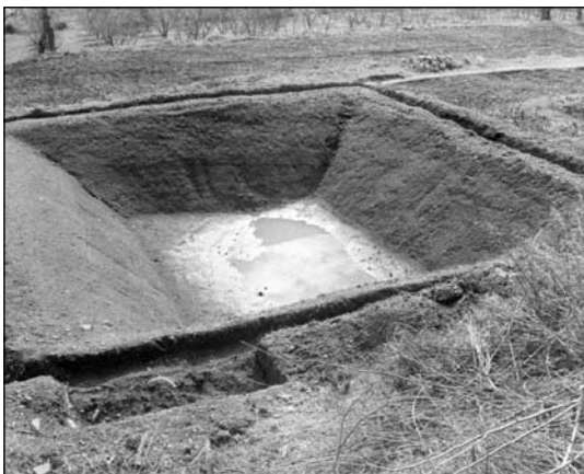
Figure 3. Construction procedure of LDPE lined farm pond
