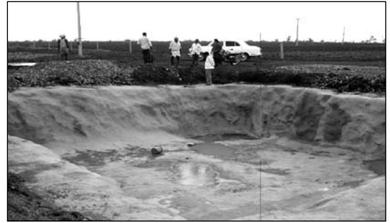
Farm pond lined with cement + murrum (1:6)
