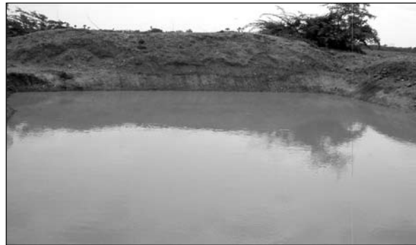
Farm pond lined with sodic soil
