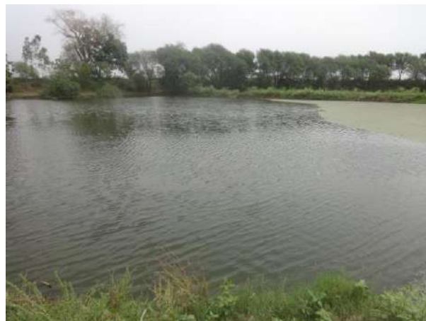
Water harvesting structure – village Nainwan
