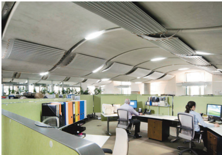
Figure 2: DesignInc, Council House 2, Melbourne, Australia, 2006, shaping and materialisation of the load-bearing concrete structure in function of reduction of the energy consumption of the building, illustrated in interior. [Source: http://www.metrohippie.com/council-house-2-council-house-1/ ]
