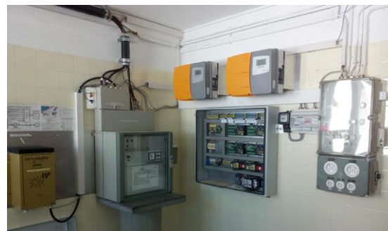
Figure 7: Modernising the high-alpine PV installation at Jungfrauoch (3,454 m asl) in autumn 2014 with new Sunpower modules.
