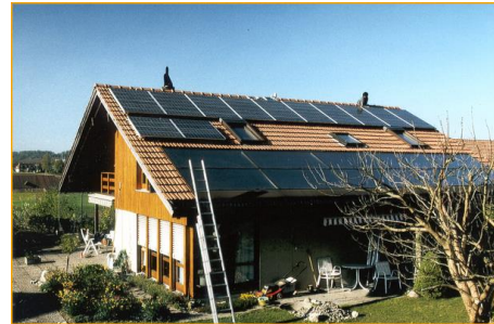
Figure 3: PV-installation at Burgdorf (540 m asl).
