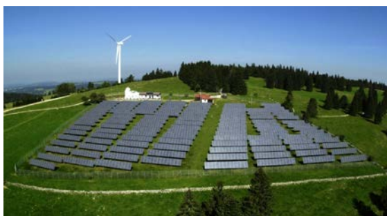
Figure 1: PV plant Mont-Soleil
