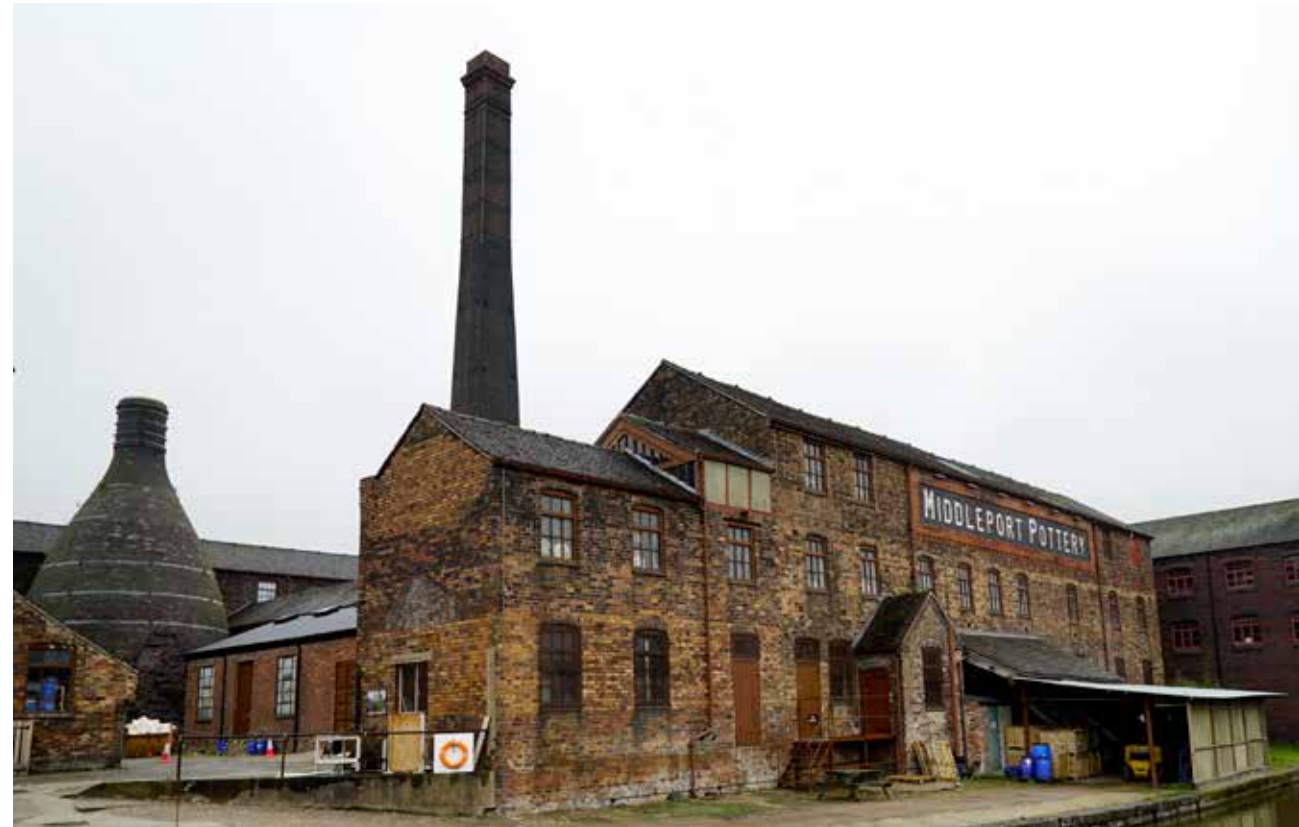
Fig 11. Middleport Pottery, recently restored by the Princes Regeneration Trust and part of Stoke-on-Trent's Heritage trail destinations
