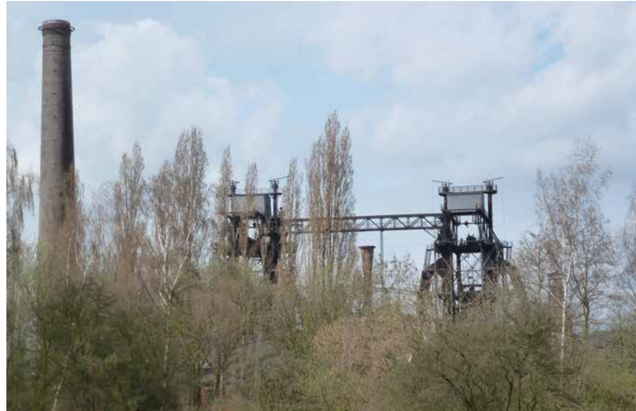
Fig. 3. Duisburg Nord Landscape Park, Germany
