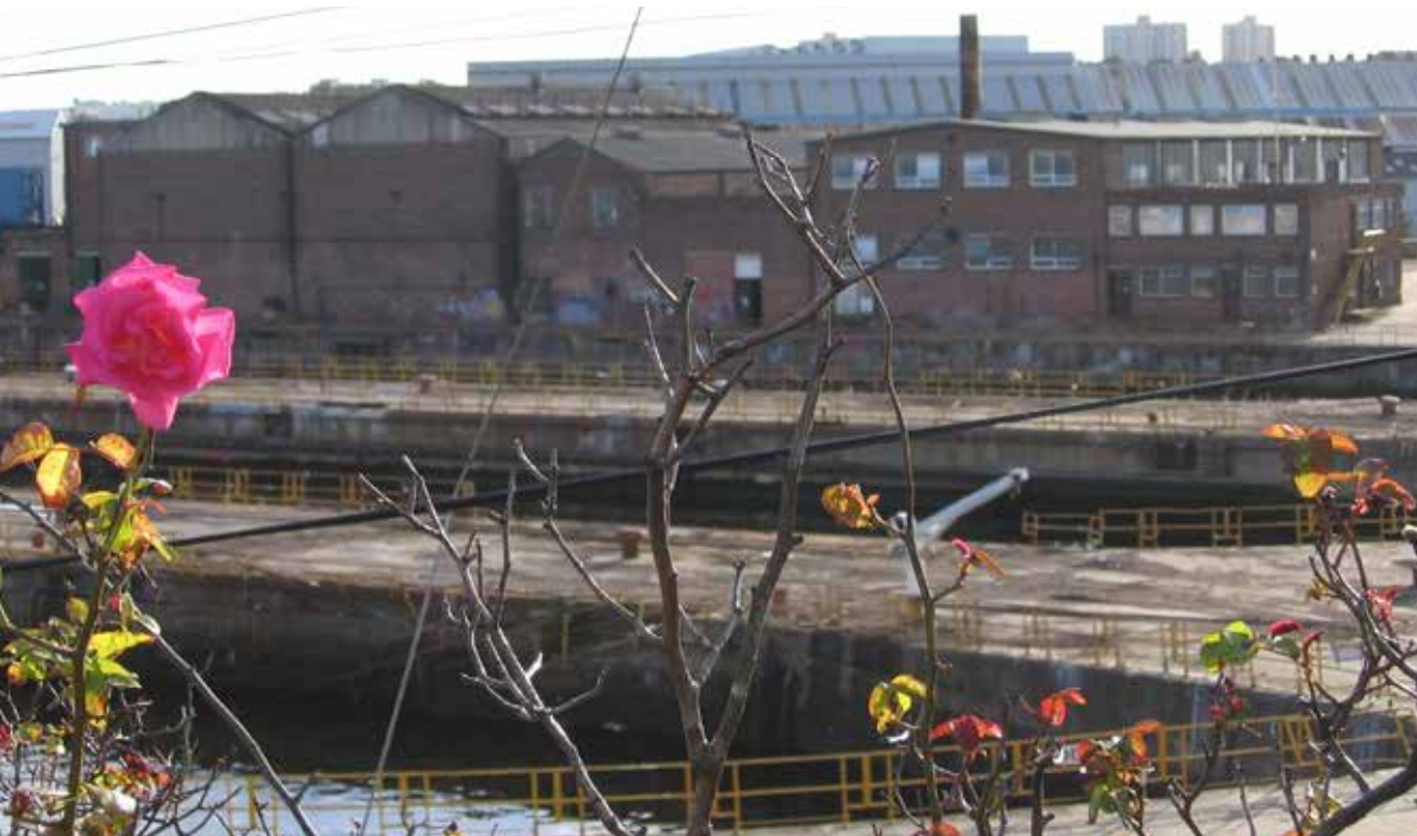
Fig. 2. Abandoned shipyard, Walker Riverside, UK, September 2005
