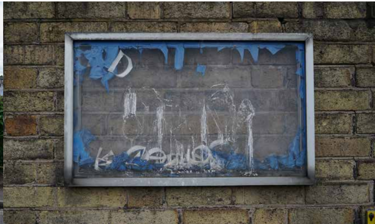
Fig. 15. Signage, former Royal Doulton site, Burslem
