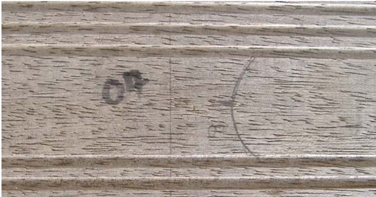
Figure 4.14 Iroko decking board untreated exposed to weathering for six months.
