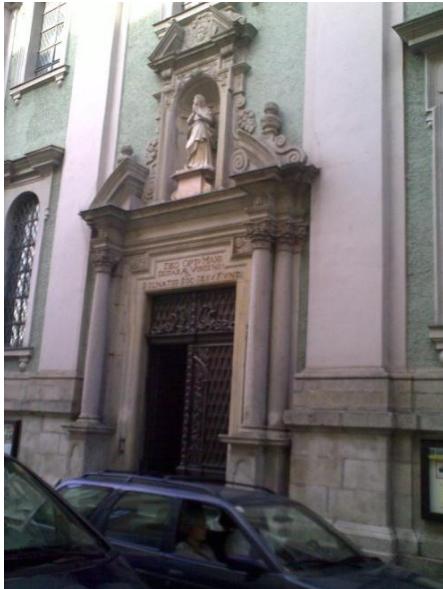
Figure 37: Church in Linz Source: personal archive
