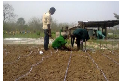
Plate 2: Installation Layout of the IDI system
