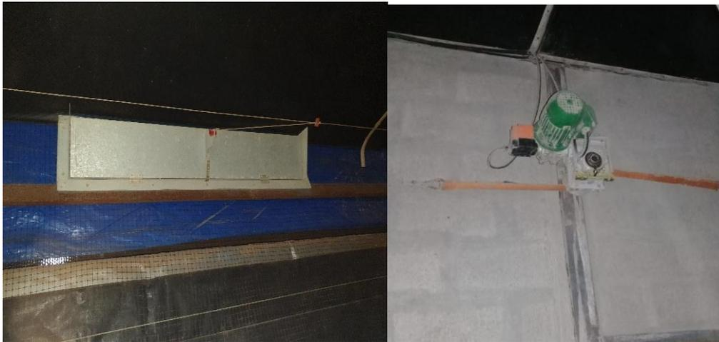
**Figura 5-2:** Inlets y Motor de Inlets
