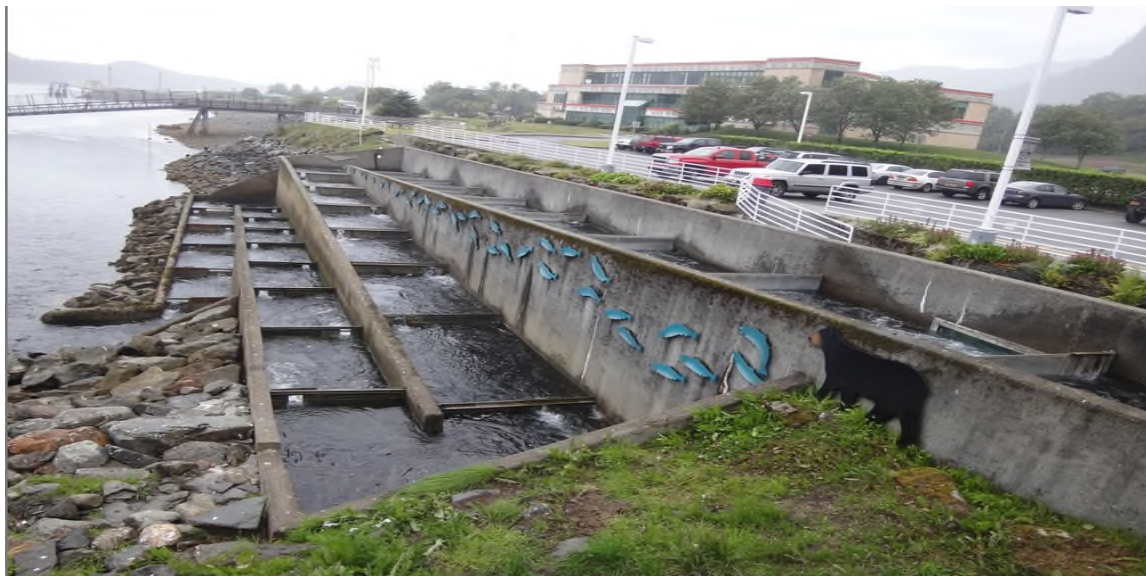
Figure 17a. Salmon ladders of Macaulay Salmon Hatchery of Douglas Island Pink & Chum, Inc. , Juneau, AK, USA. (Credit: LK Wang and MHS Wang)
