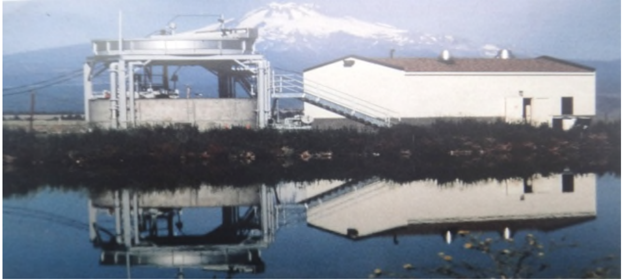
[ Insert Figure 42. Full-scale double DGF-DGFF (or DAF-DAFF, or Supracell-Sandfloat) system ]
