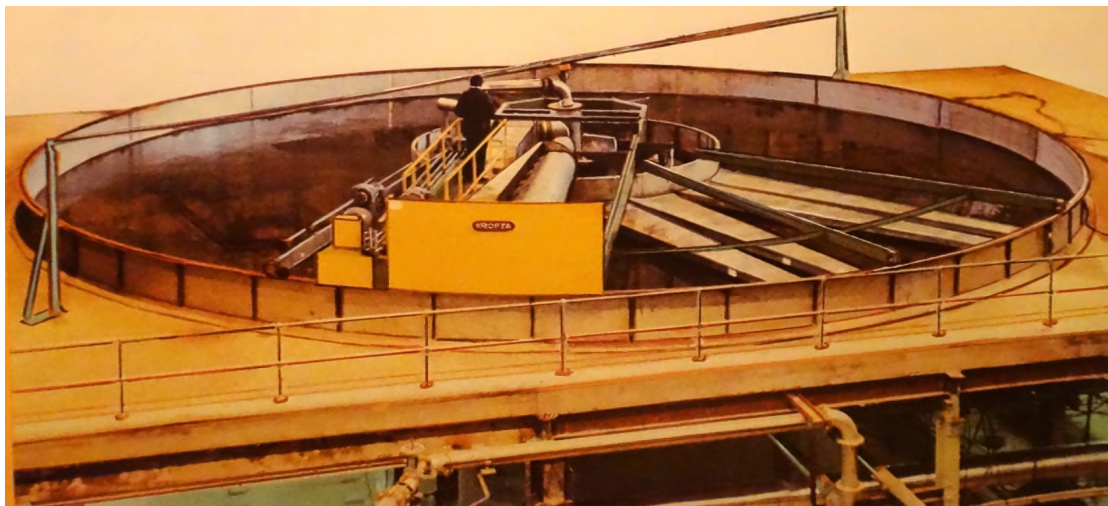
[ Insert Figure 19. A high rate dissolved gas flotation clarifier in UK (Supracell 62; tank depth = 750 mm; flow = 35.2 \text{m}^3/\text{min} ; diameter = 62 ft = 19,900 mm) ]
