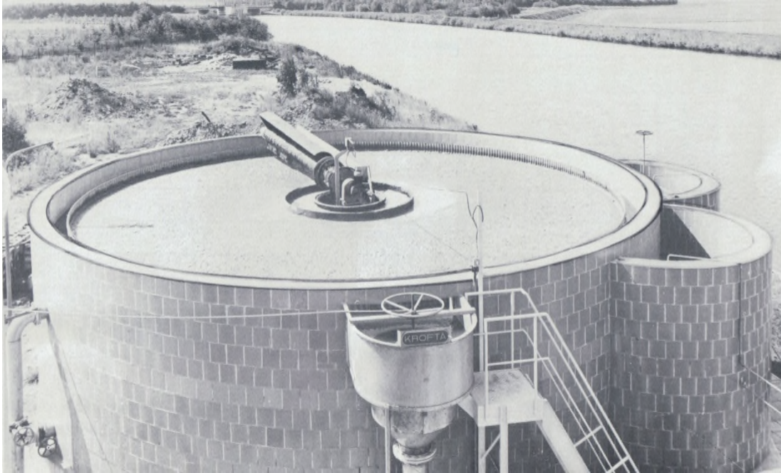
[ Insert Figure 26 . Construction of Sedimentation-Flotation Clarifier (SDF-36FT) in Acid-Resistant Tiles (Holland) ]
