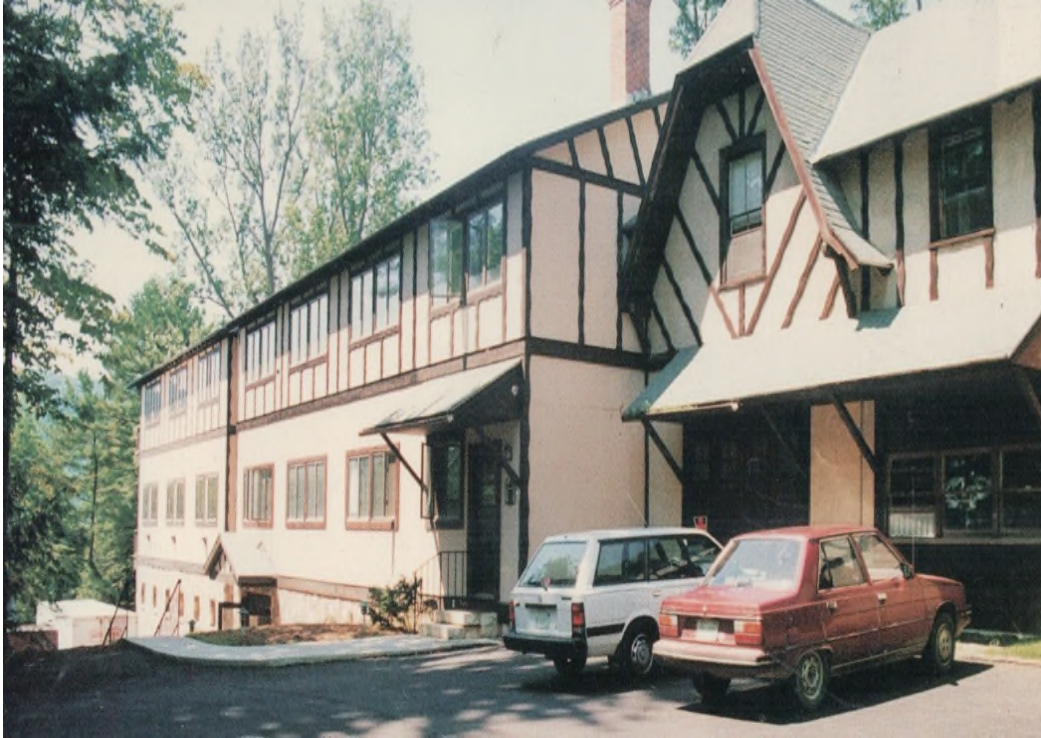
[Insert Figure 1. Lenox Institute of Water Technology (LIWT), Massachusetts, USA]
